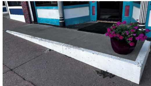
Some entries have safety rails or painted edges and barriers to warn pedestrians of the drop-off. When sidewalk streetscaping occurs, it should incorporate a solution to business entries that provides a safer environment. Until then, painting all drop-off edges is an immediate need and minimum recommendation.
