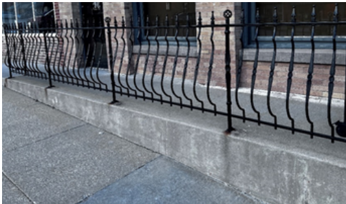
Some entries have safety rails or painted edges and barriers to warn pedestrians of the drop-off. When sidewalk streetscaping occurs, it should incorporate a solution to business entries that provides a safer environment. Until then, painting all drop-off edges is an immediate need and minimum recommendation.
